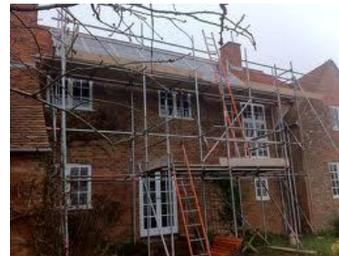
Local scaffold companies x 5
