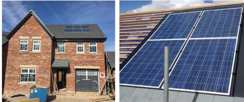
In Roof Silver Frame Polycrystalline Panels
