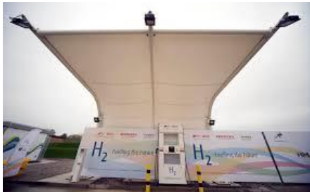
Swindon solar powered refuelling station
